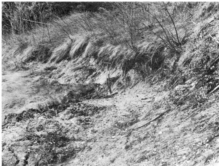
Fig. 18. Lite teleras i silt ved Kalvskinn (744 109). Foto P.A. Kjærnes. Small slide caused by thawing of ice in silt at Kalvskinn (744 109).
