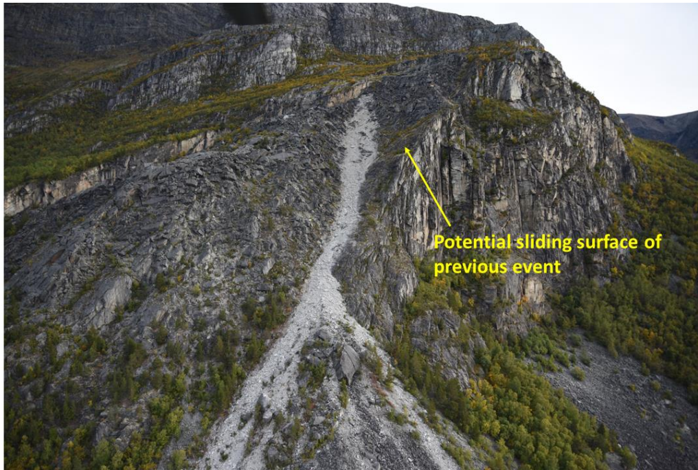
Figure 12) The main body of the strongly deformed unstable slope (to the left) and the underlying massive, undeformed bed rock below a failure surface. This failure surface might have formed during a large event or due to continuous rock fall from the unstable rock mass. The trace of the October 12, 2019 rock fall marks the limit between the unstable rock mass and the failure surface. The back scarp of the unstable rock mass is visible as a bright pink coloured rock band in the background.
