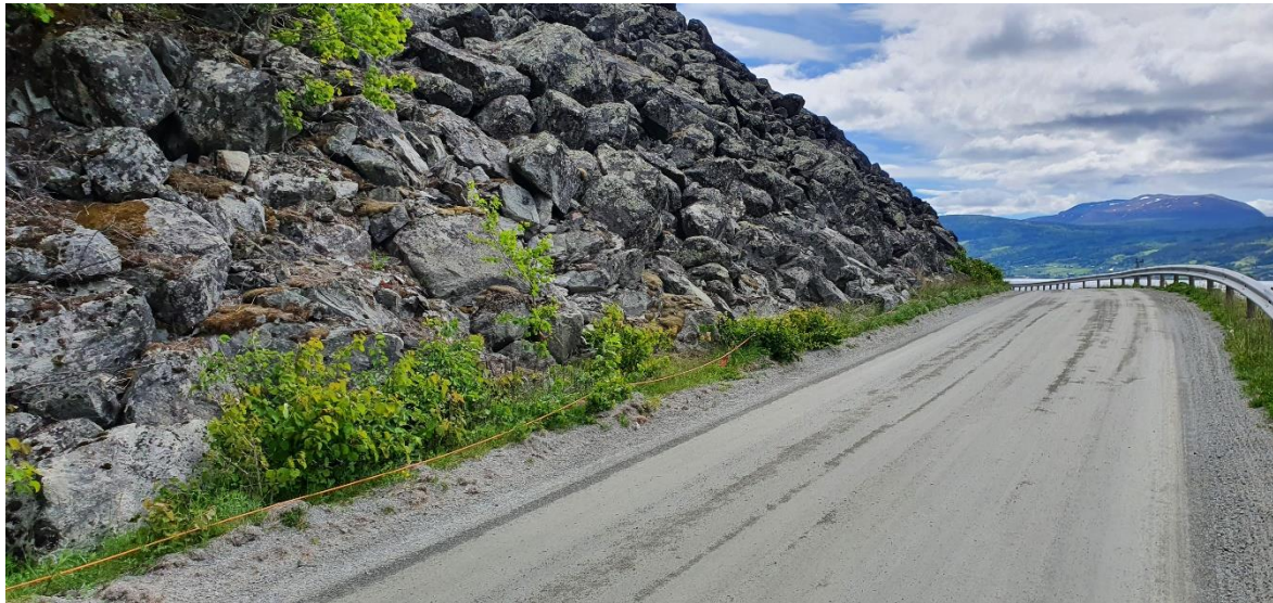
Figure 19) Cable set up between road and scree.
