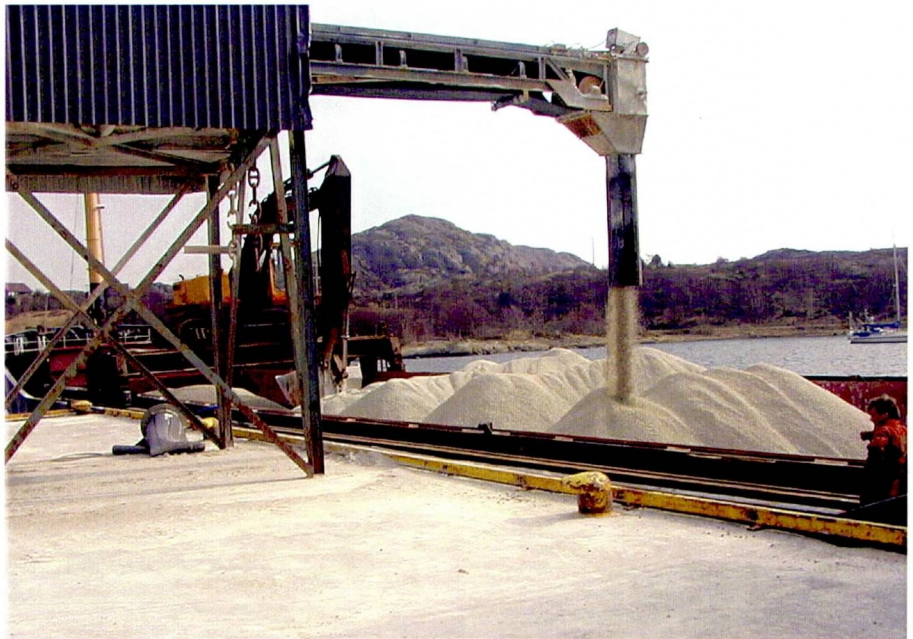
The Norwegian Edelsplitt KS plant at Hellevik in Eigersund, Rogaland, where white anorthosite is produced for use in asphalt and ceramics.
