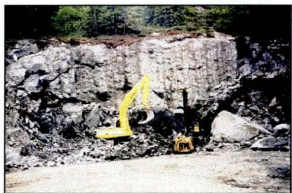
Development of New Access Tunnel
