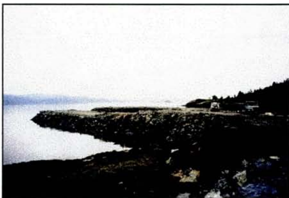
New Port Facility
