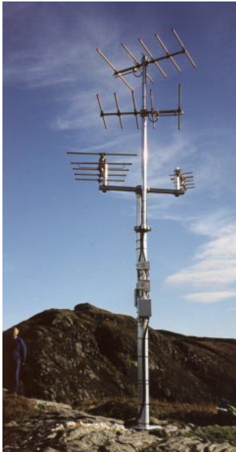
Fig. 7.1.3. The receiver mast at the central station, Bremanger.
