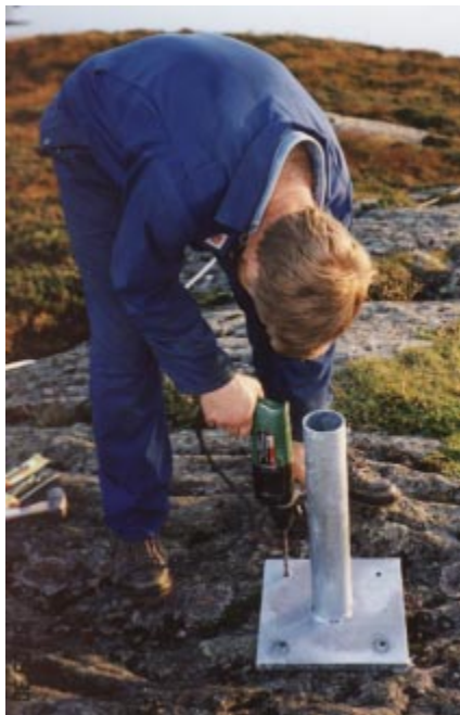
Fig. 7.1.5. Drilling the foundation for one of the masts.
