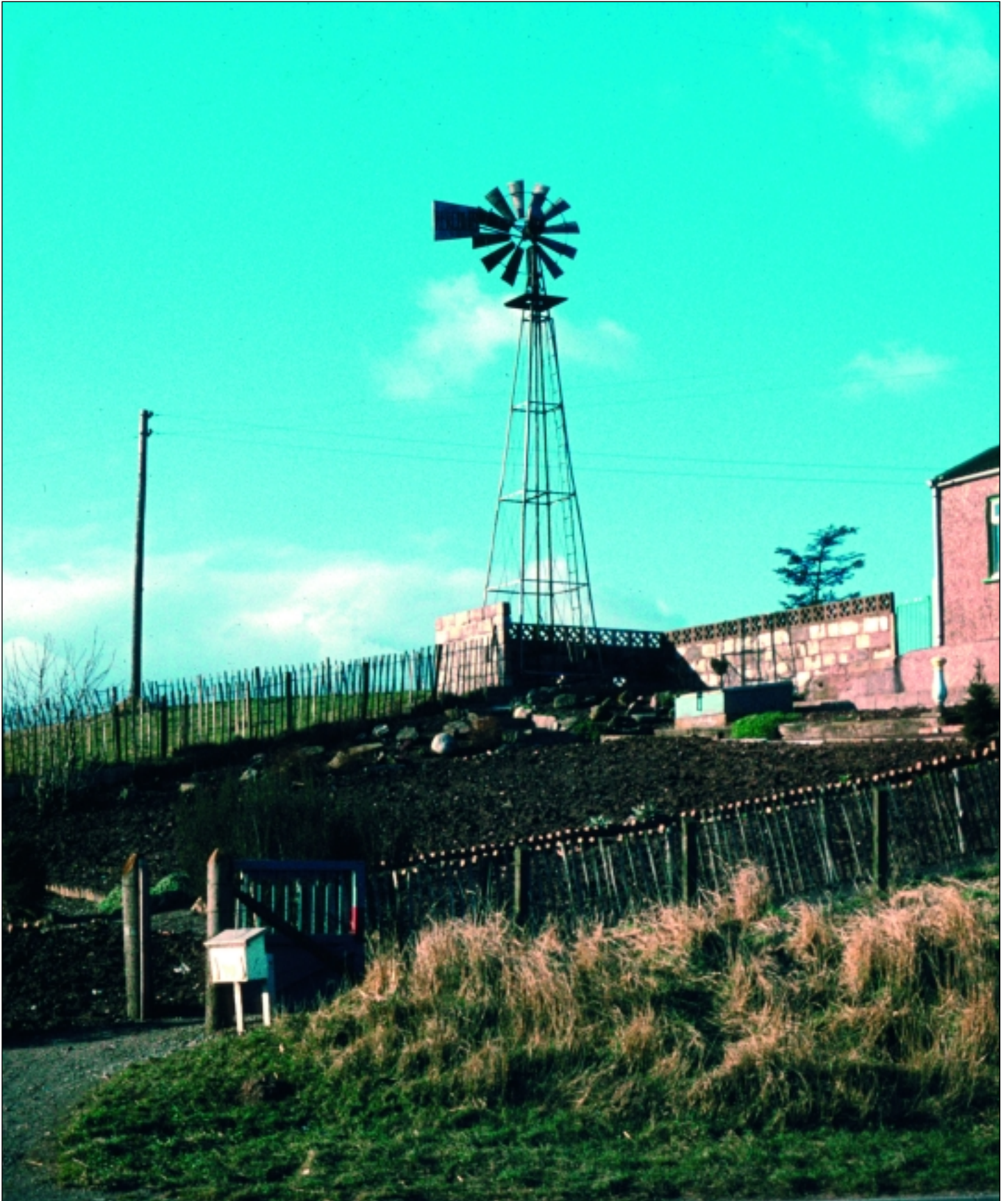
Figure 19. A wind-pump used for pumping groundwater at Stonehaven, Scotland (photo: Nick Robins).
