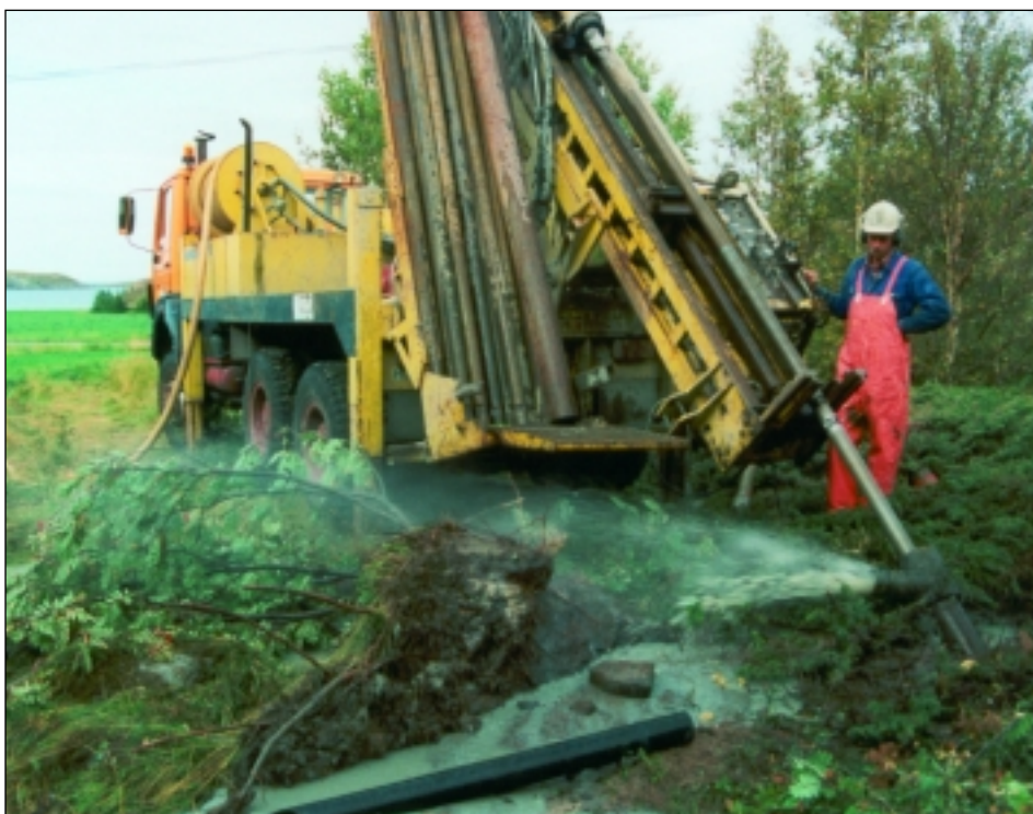
Figure 16. (a) A modern downhole hammer rig drills a deviated borehole in the gneisses of Flatanger municipality, Norway. (b) Schematic diagram showing optimum borehole orientation to meet a fracture zone. The angle \alpha (borehole fall) should be such as to meet the fracture zone at a depth of some 40 - 50 m. The lower the angle \beta , the longer the portion of the borehole within the zone, but the greater the angle \beta , the less the danger of missing the zone altogether.
