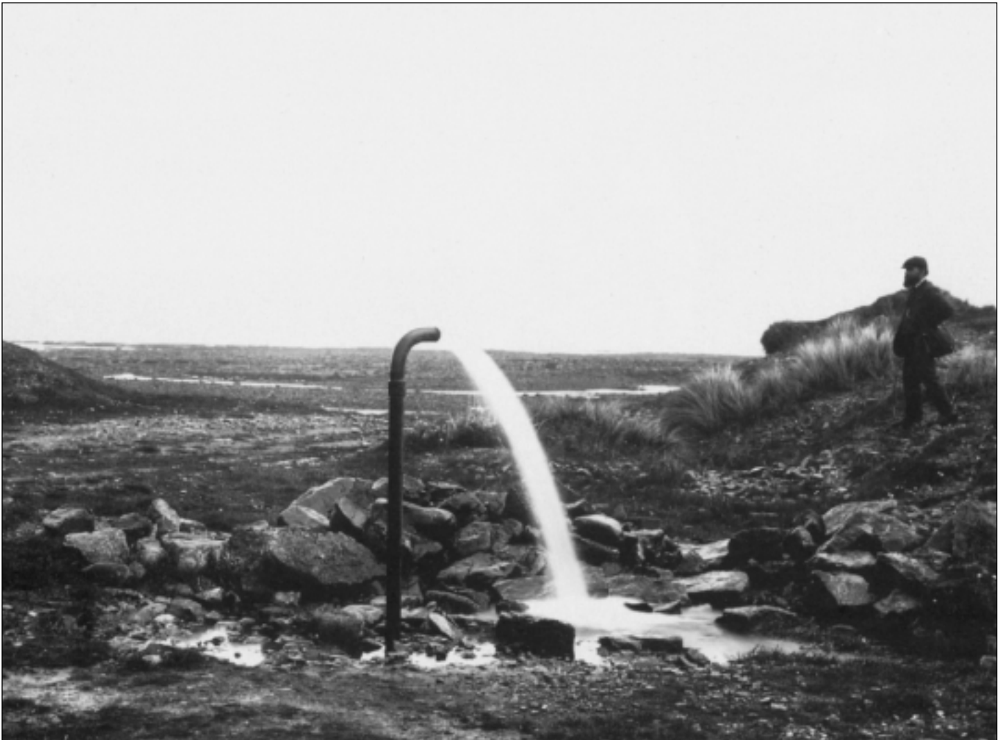
Figure 2. (c) an artesian (overflowing) borehole in Carboniferous rocks at Catcraig, near Dunbar, Scotland. The photo features the geologist C.T. Clough and derives from c. 1908 (after Robins 1990). Printed with permission from British Geological Survey.
