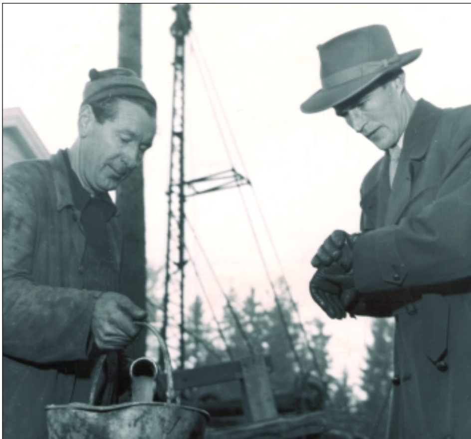
Figure 21. (a) An elegant Steinar Skjeseth assists a driller in measuring water flow during the test-pumping of a well.
