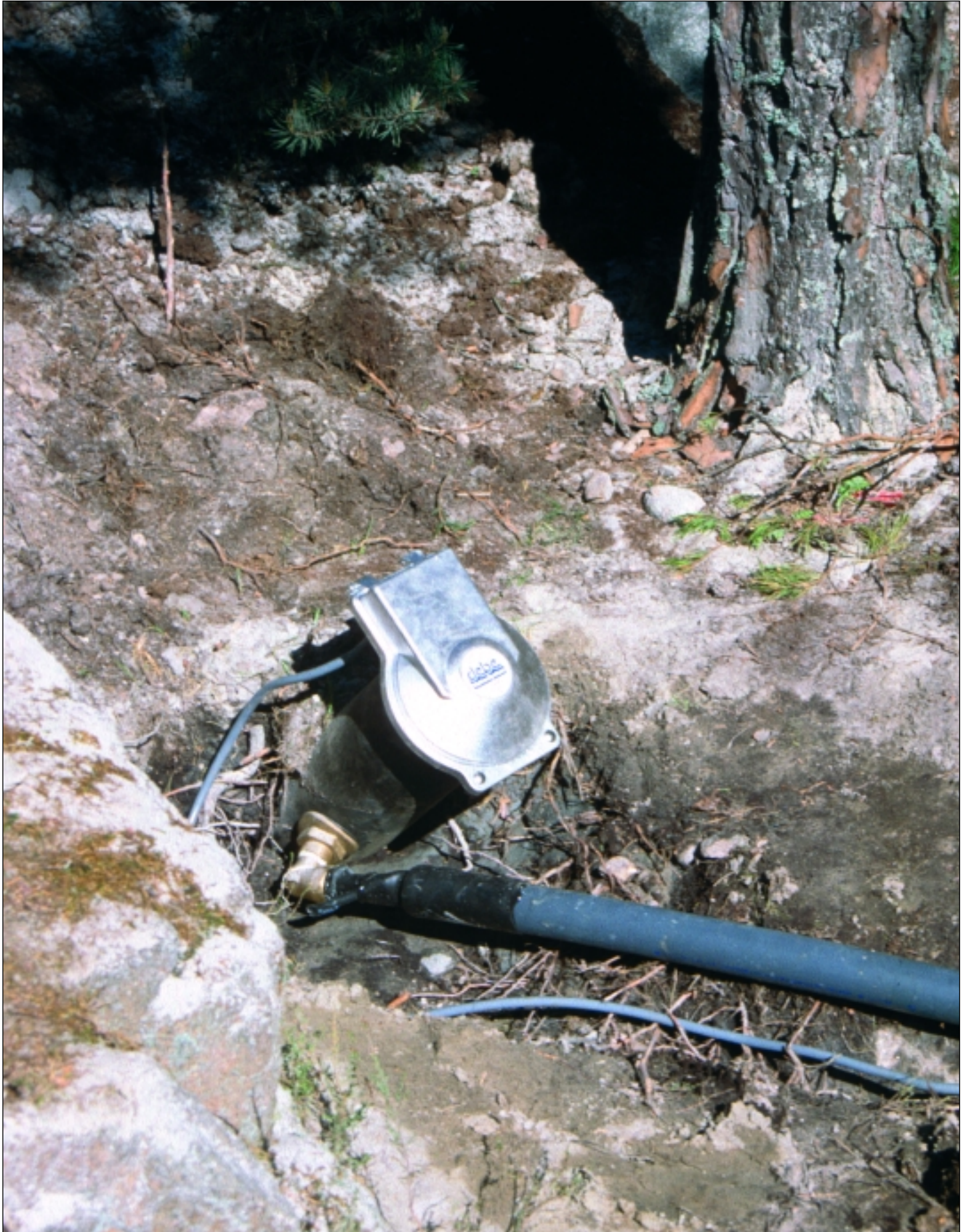
Figure 2. (d) A modern, angled borehole in granite, Hvaler Islands, Norway (photo: David Banks).
