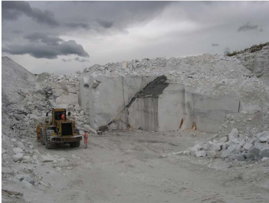
Figure 6: Attempt at re-opening dimension-stone quarry in white dolomite at Løvgavlen, Fauske.
