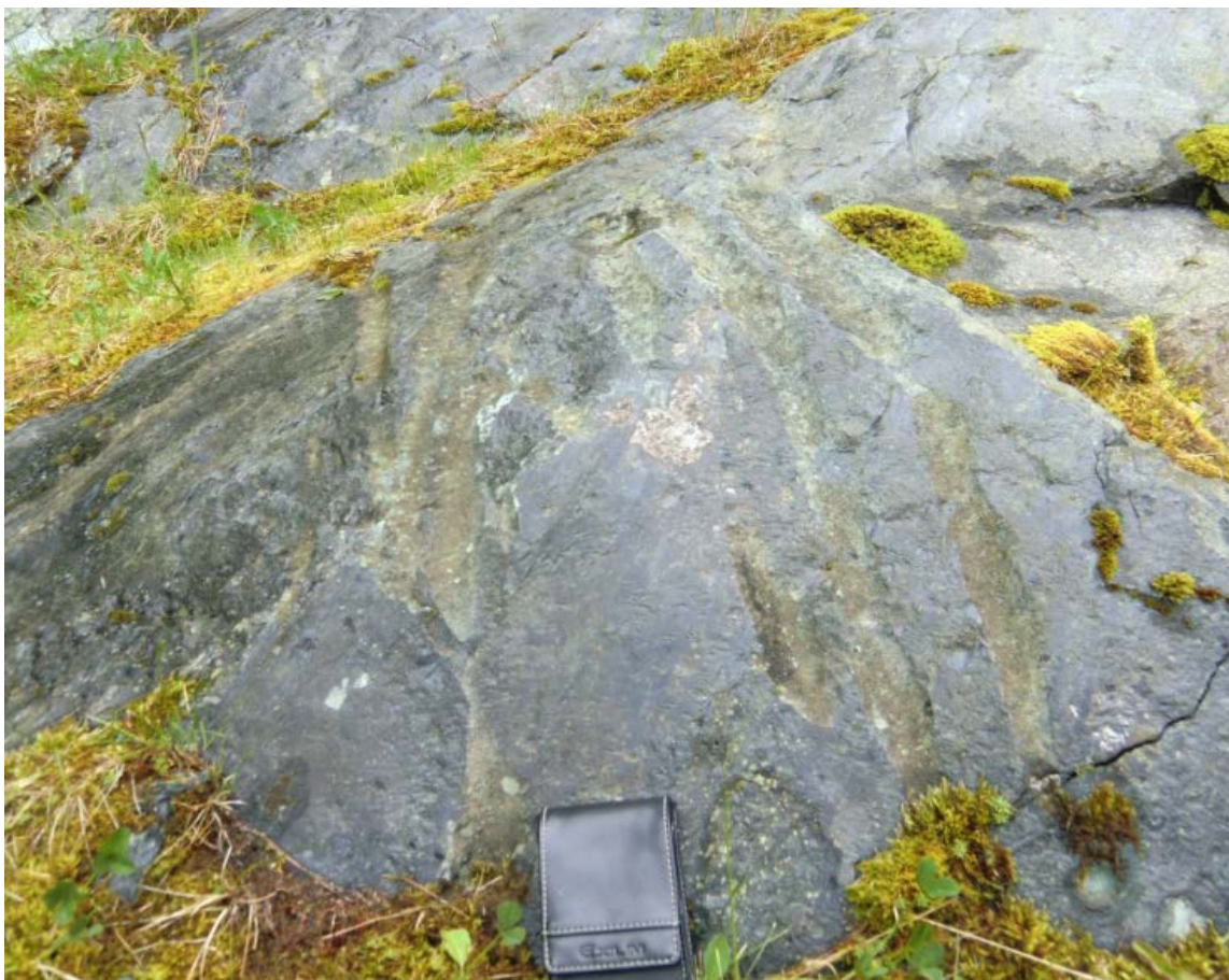
Figur 37: Dype riss i berget.
