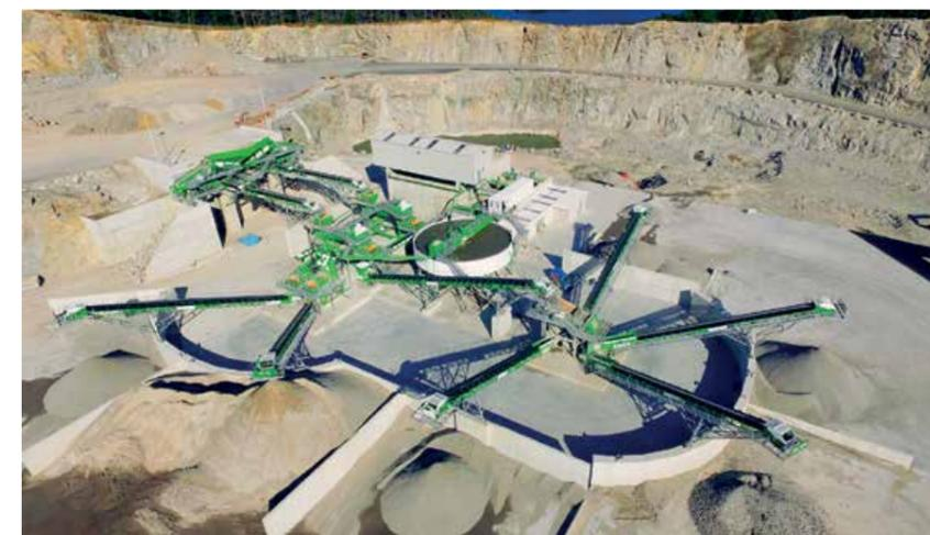
The aggregate plant at the Velde AS stone quarry is integrated with the concrete and asphalt station and a modern recipient plant for construction materials. This reduces the transport needs and the environmental impact. Foto: Velde AS
