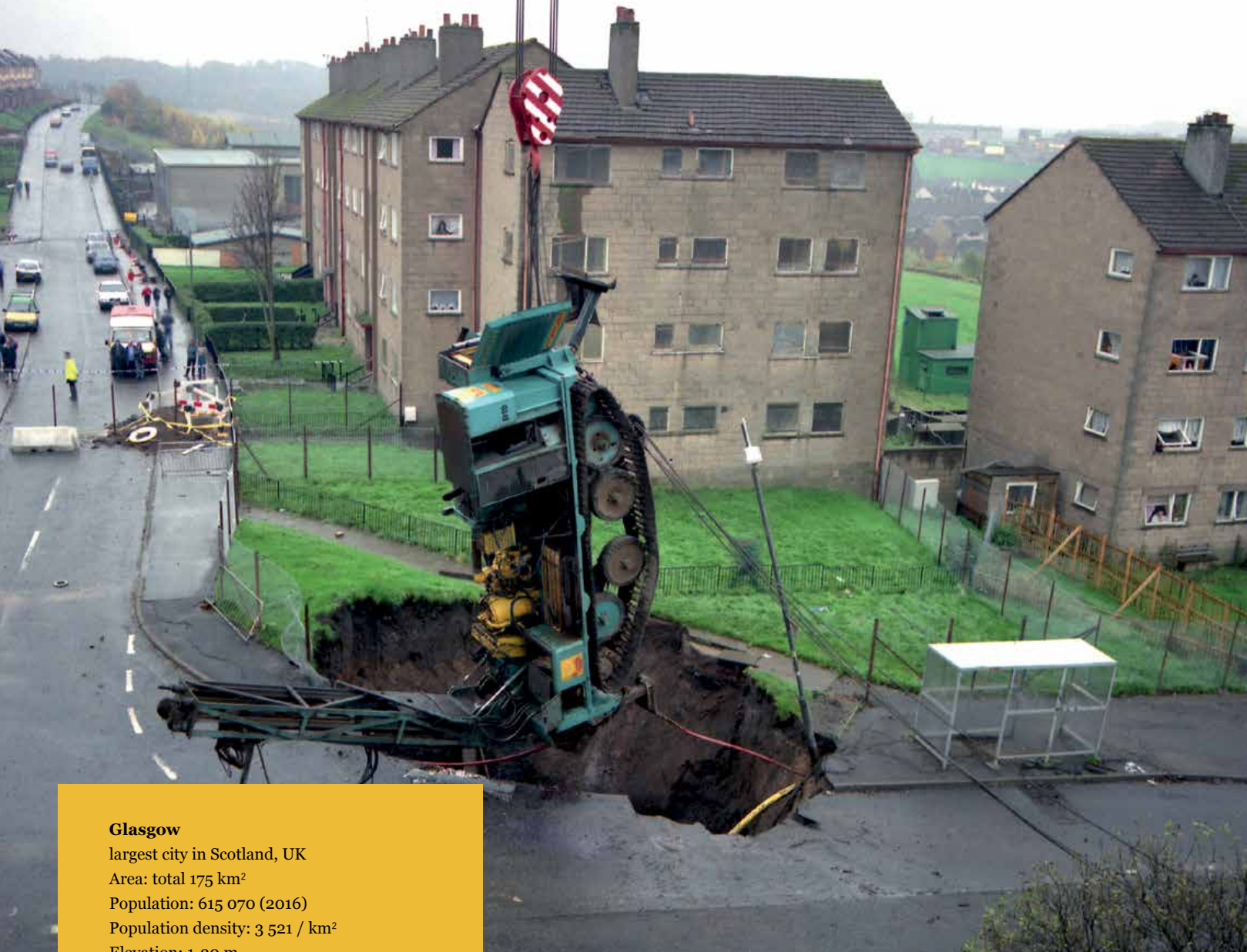
A catastrophic collapse of an abandoned mineshaft. Photo: BGS
