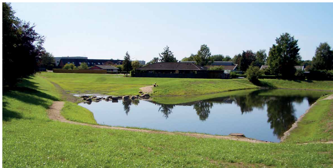
A Park with retention basin, as a measure to deal with flooding of the neighbourhood Sanderum. Once an area with seven private properties and homes, now functions both as recreational area and a storm water basin. Photo: Johan Linderberg. For more info see: www.klimatilpasning.dk
