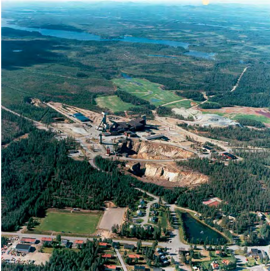
Figure 24. Aerial photo of the Kristineberg deposit with open pits and the head frame. Copyright: Boliden Mineral AB.
