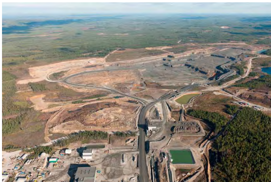
Figure 61. Talvivaara mine site in 2010; view to the SE. The extent of the excavated area is 0.7 x 2.5 km. Photo courtesy Talvivaara Mining Co.
