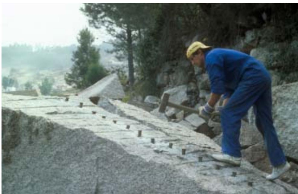
*Worker using short plugs for wedging granite block in Vigo, Spain.*
