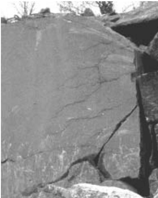
*Figure: damages (cracks) from blasting*
