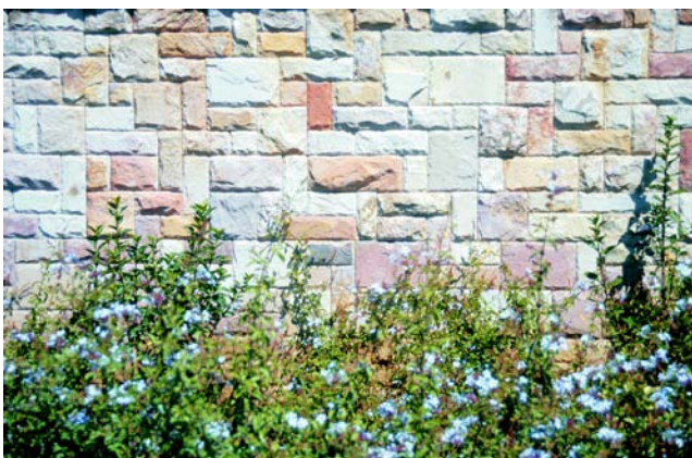
Fig. 13. Wall clad with the Ambo sandstone, Hotel Sheraton, Addis Ababa.
