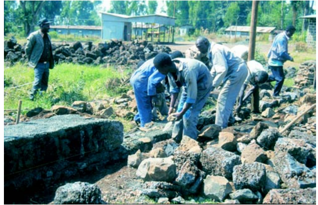
Fig. 14. Wall construction with vesicular basalt near Debre Markos.
